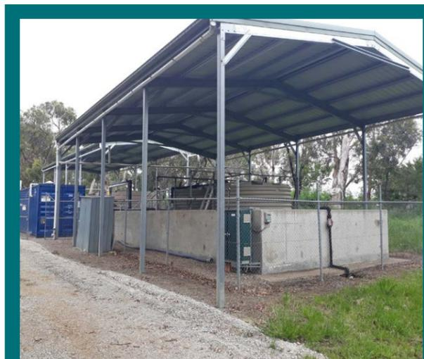
Coldstream leachate plant – the plant processes leachate liquid collected from the landfill for disposal into the sewer system. This is important to ensure that the liquid does not contaminate local groundwater and the surrounding environment.
